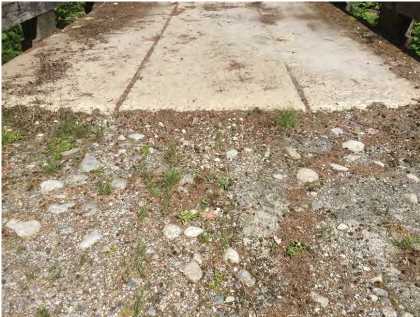
Left approach requires 150mm gravel depth
