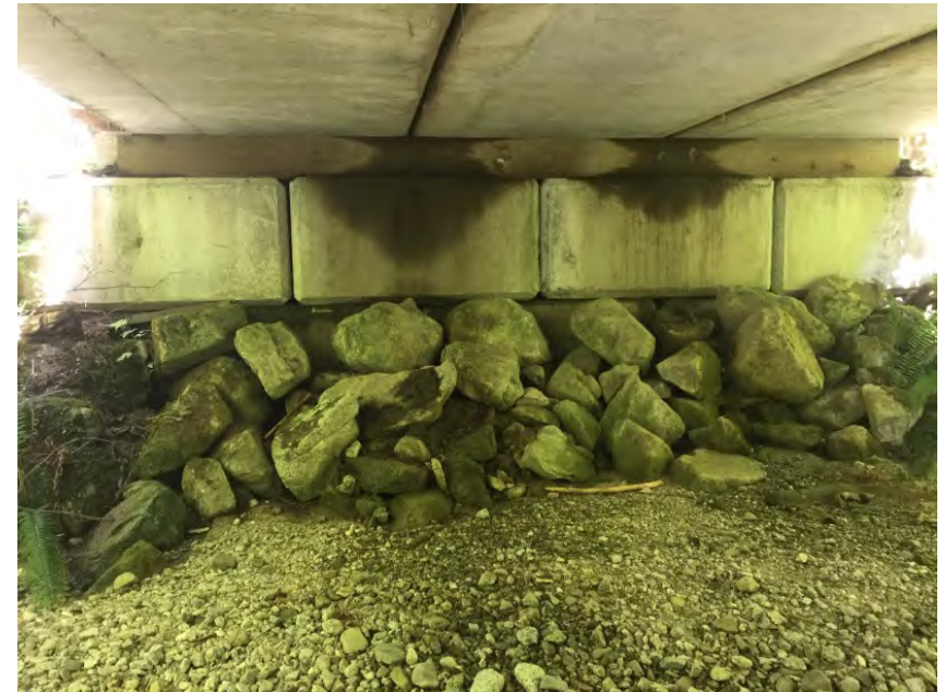
Right Bank Abutment when facing downstream
