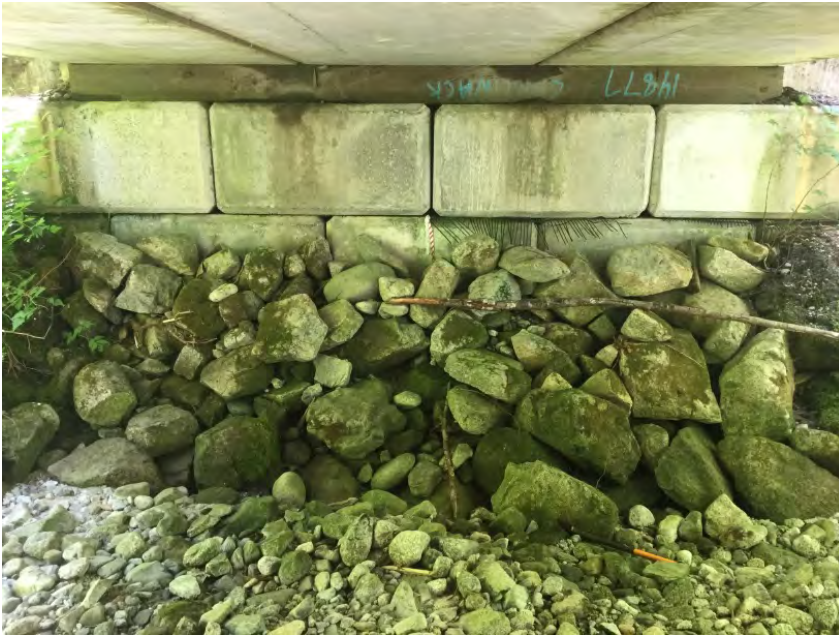
Left Bank Abutment when facing downstream
